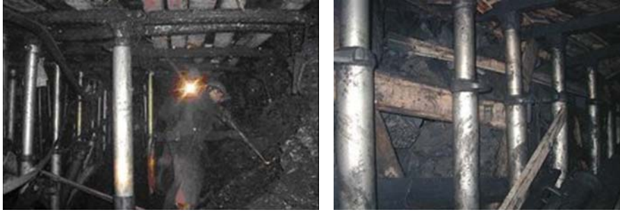
FIGURE 1: Mining labour supported by individual hydraulic props.
