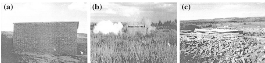
Fig. 2.31 Deconstruction/damage of n -butyl nitrate for brick structure buildings, a before explosion, b in explosion, c after explosion
