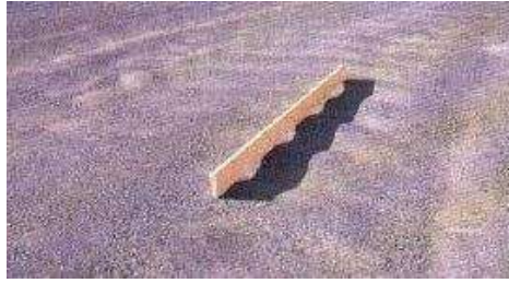
Gambar 2.4 Keriting ( Corrugation ) (Sumber : Bahlawant, 2011)
