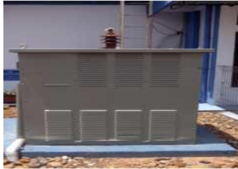
Gambar 2. 15 Neutral Grounding Resistance (Pratomo et al., 2022)
