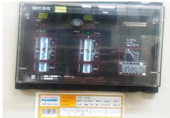
Gambar 2. 12 Relay Over Current (Sumber: PT. Indonesia Power)
