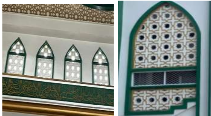
Gambar.7 Ventilasi Masjid Al-Munnawar
